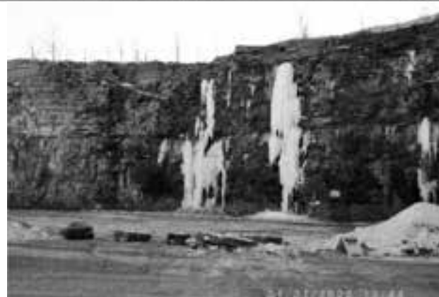
A miner was severely injured while working near the base of an approximate 65 ft. highwall. The miner was struck by loose, fractured and overhanging rocks.
